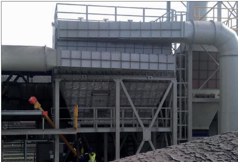
**Fig. 2** Herding MAXX filter series for large volume flows
