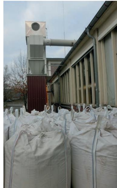
**Fig. 5** Herding filter system with clean air recirculation into the production facility for technical ceramics
